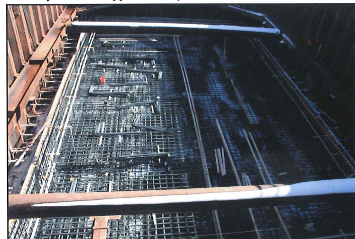
Rebar in place for Mountain well improvements.
