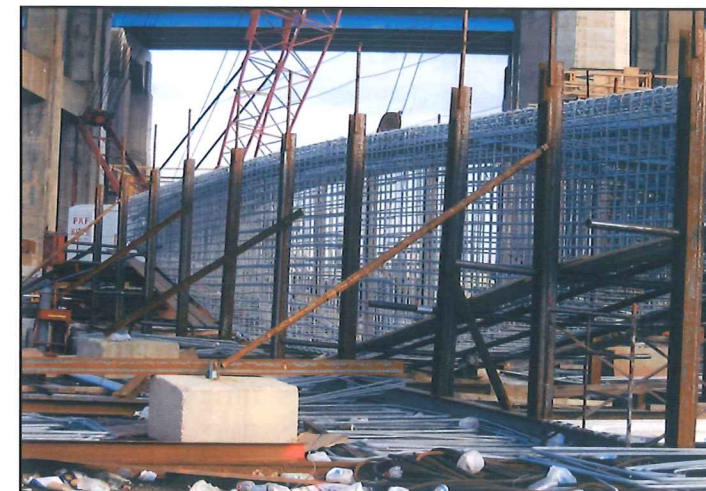
Rebar installed for the Driscoll Bridge pier caps.
