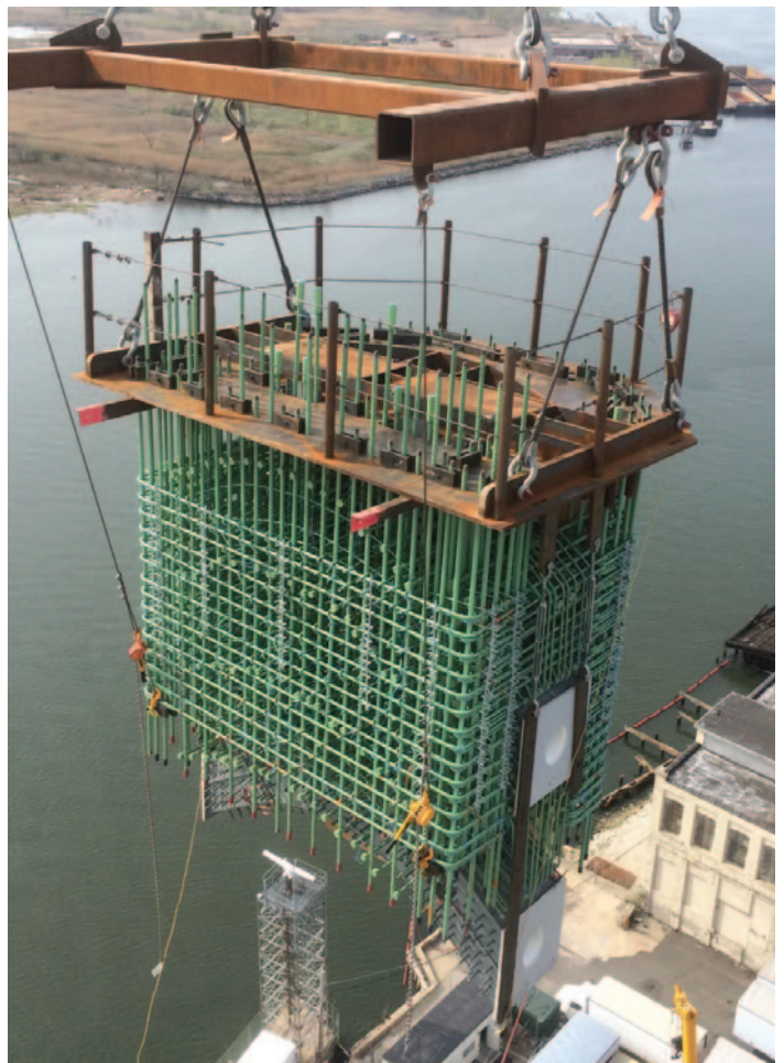
Goethals Bridge NJ Main Span & Approach (5,600 tons rebar)
