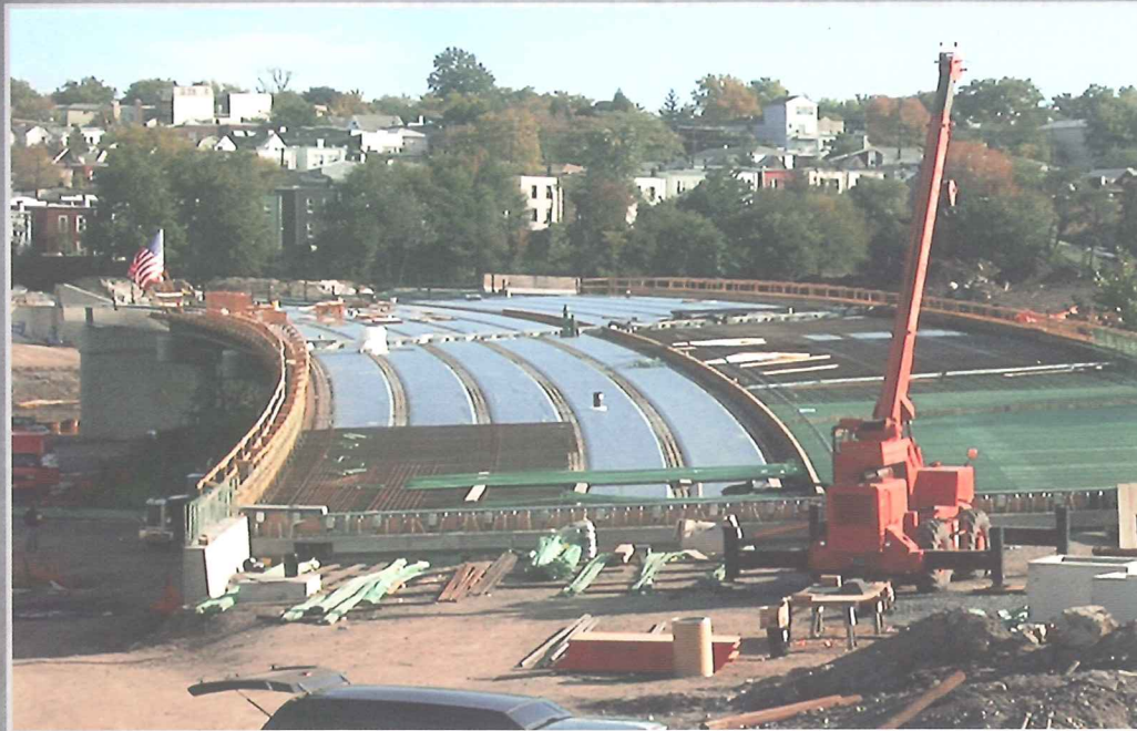
Hudson-Bergen Light Rail Project. Secacus road separation over Routes 1 and 9
