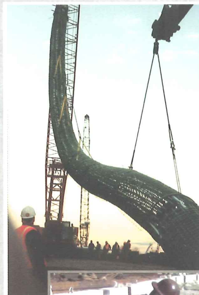
Installation of 100 ft. long caisson cages on the Route 9/Bass River Project in New Gretna, NJ.
