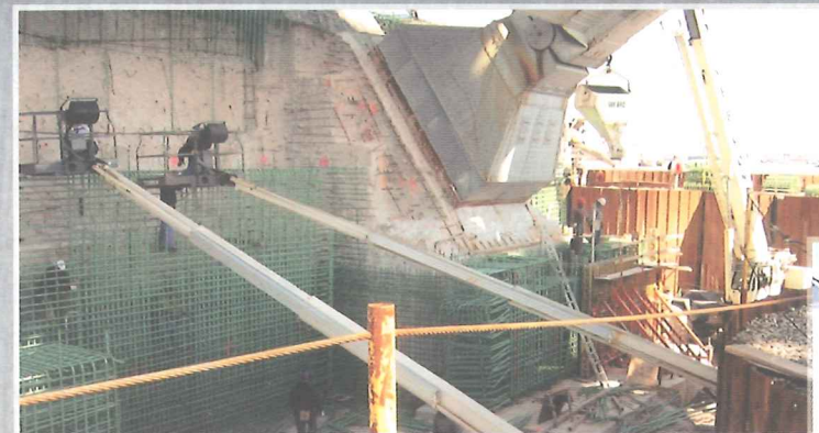
Reconstruction of the Bayonne Bridge NJ abutment
